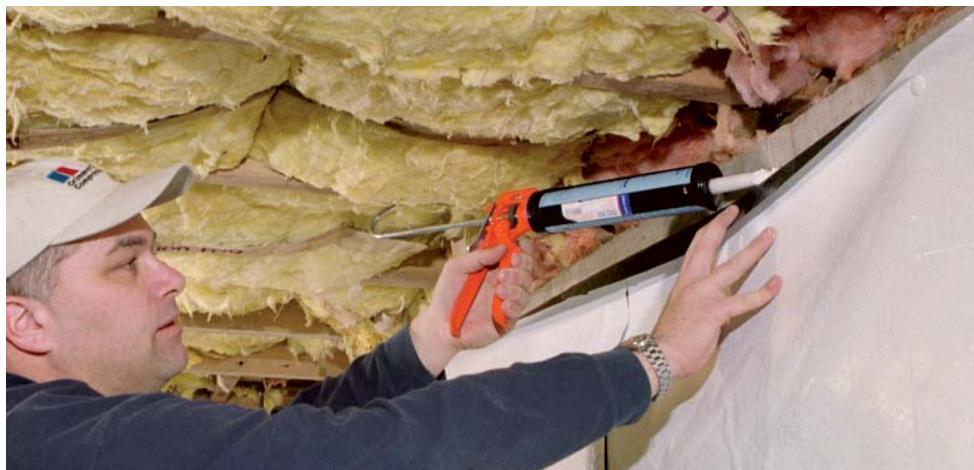
Seal the liner to the foundation with polyurethane caulk.
