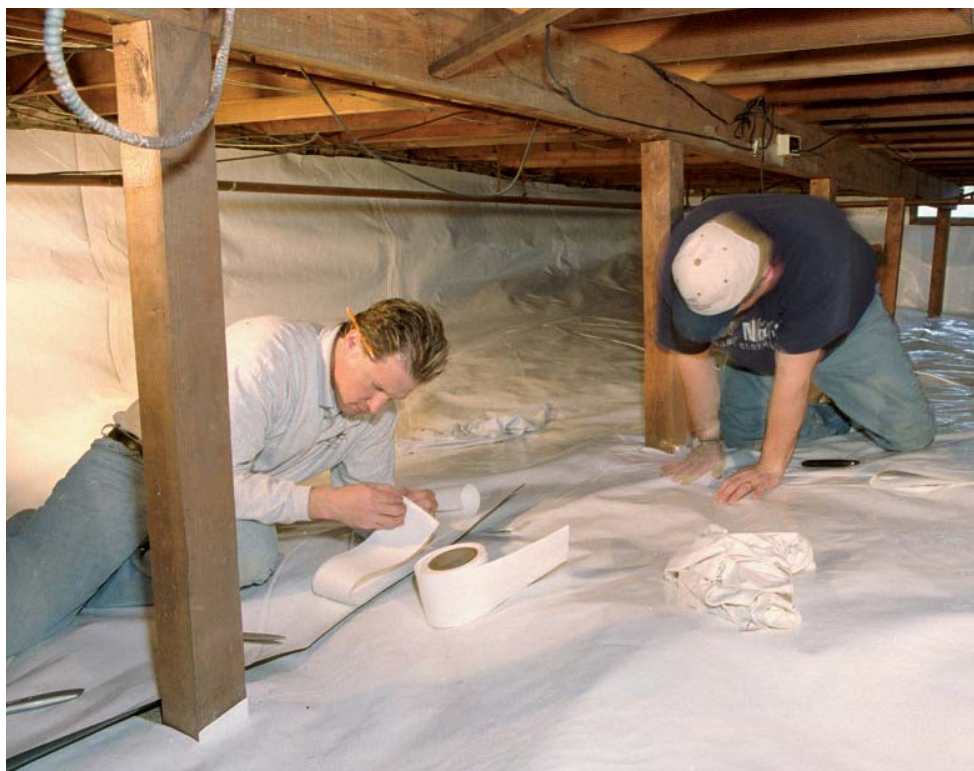
Seems like a single sheet, but it's not. Overlapping seams of the liner sections are sealed with caulk and matching tape for a seamless barrier.
